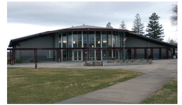
New Performing Arts Building (2003)
